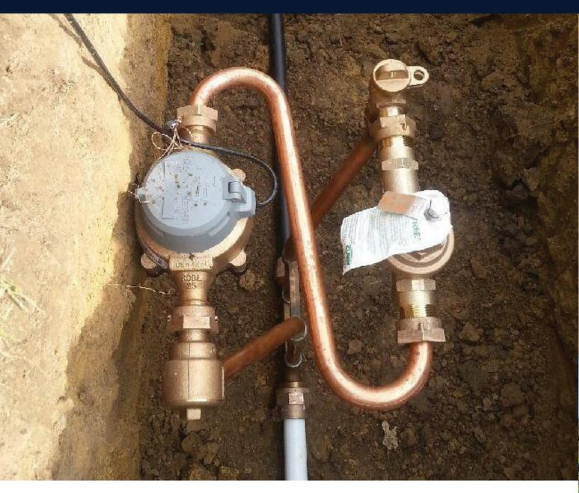
Declining meter accuracy can be an unfortunate side effect of aging water infrastructure. Over time, some mechanical devices are subject to wear, which in turn may affect their ability to accurately register flow. Consequently, this can adversely impact billing and lead to a loss in revenue.
