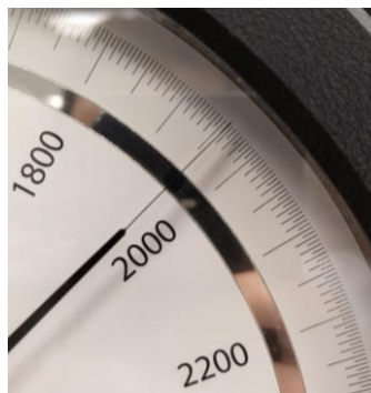
Figure 16: The indication is offset from 1950 PSI after pressurizing to span.
