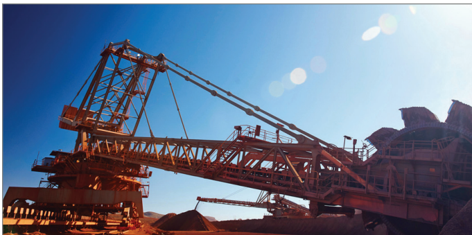
Figure 2. A long-haul conveyor moves materials from the pit to the processing plant.
